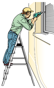
Figure 2b Correct - steps facing work activity
